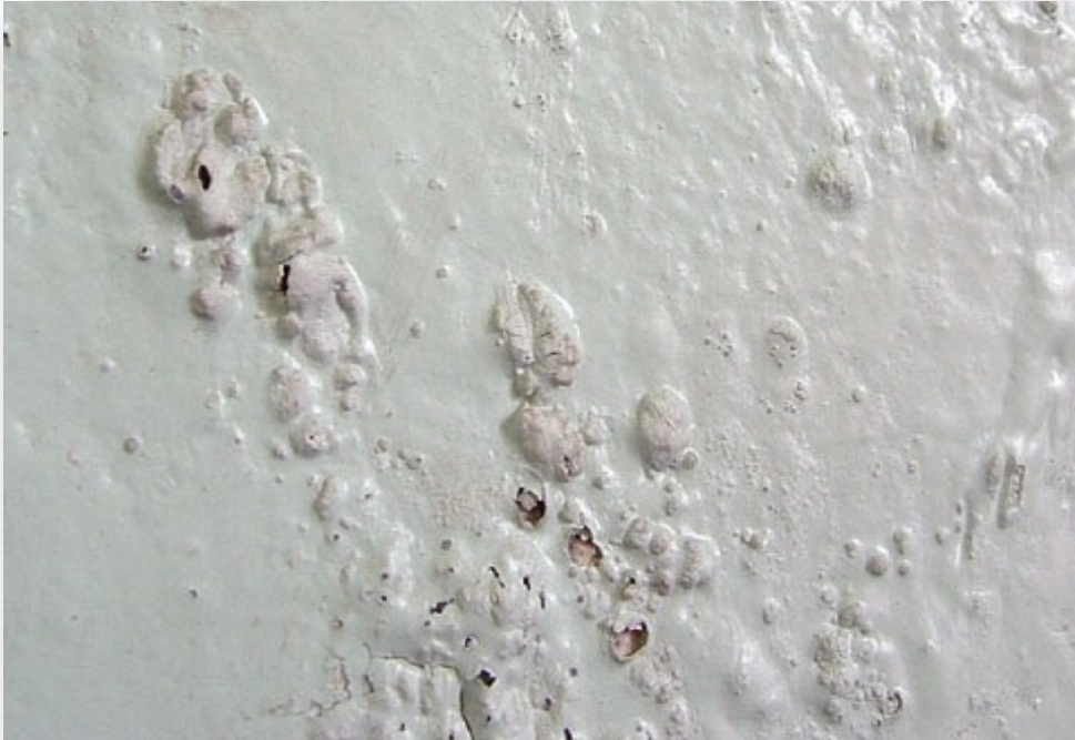
Causes Blistering of Paint
