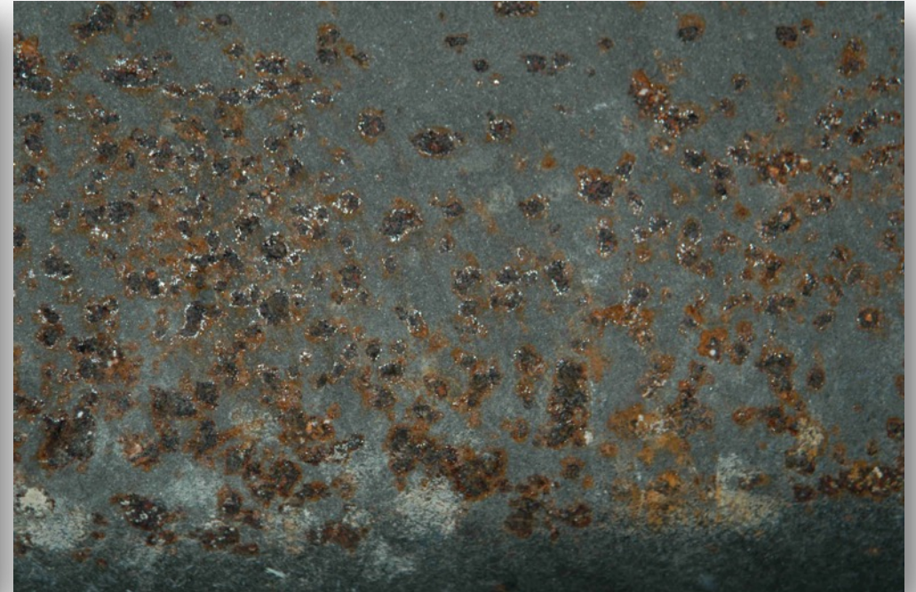
Corrosion of Metals
