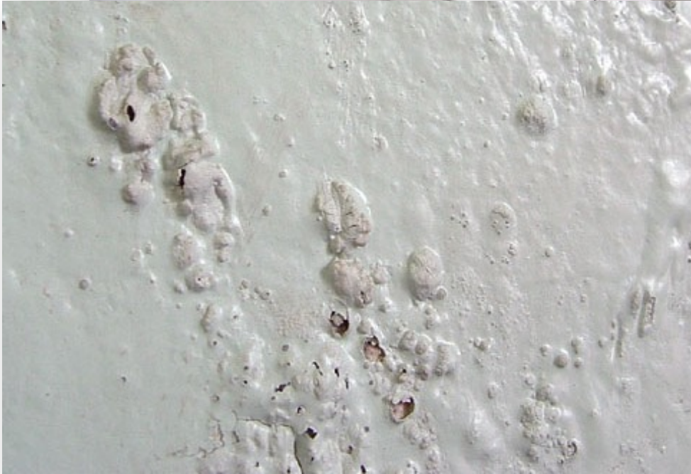
Causes Blistering of Paint
