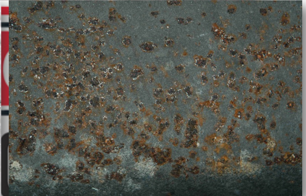
Corrosion of Metals
