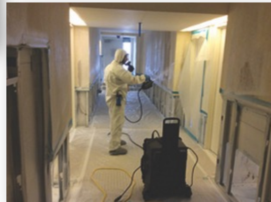
SteraMist™ Surface Unit used to treat mold in a Orange County hotel
