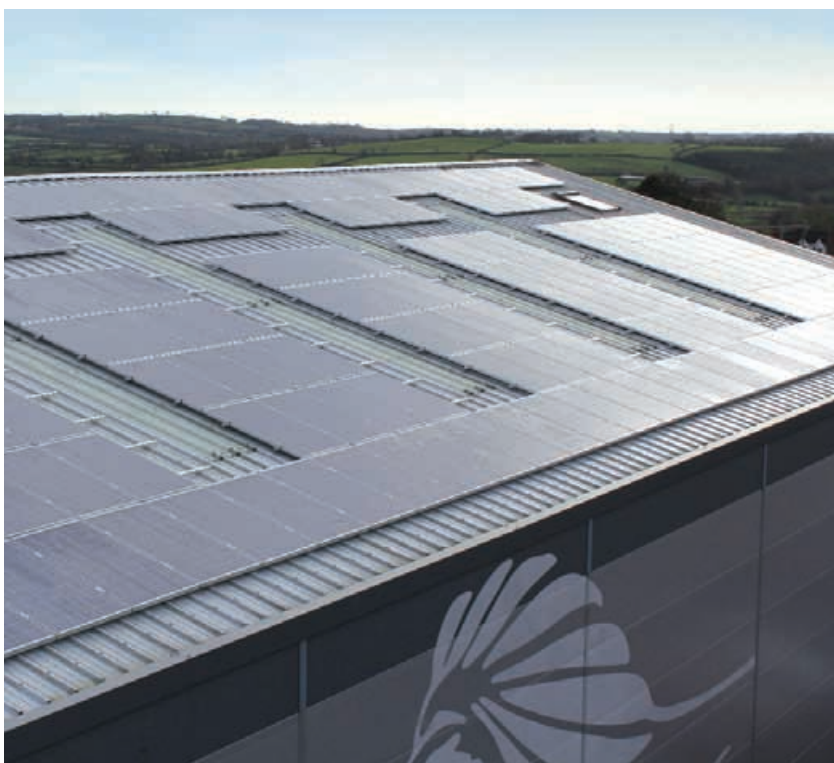
Solar Photovoltaic panels on the Kingspan Group facility at Kingscourt, Ireland.
